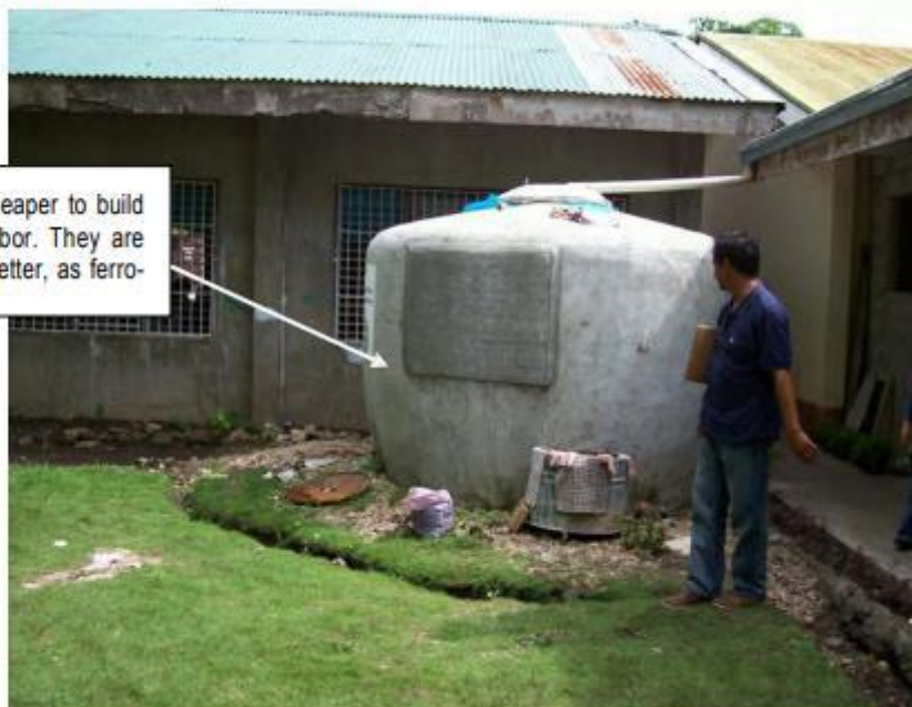
Ferro-cement water tank for rainwater collection
