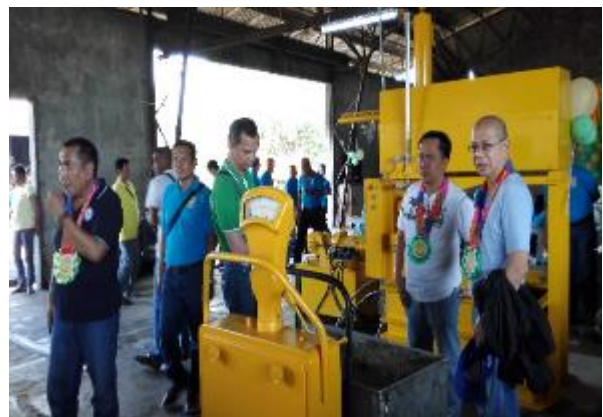
Upgraded processing plant of United Workers ARB MPC, located in Menzi, Isabela City, Basilan. Funded by LBP
