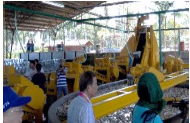
Upgraded processing plant of United Workers ARB MPC, located in Menzi, Isabela City, Basilan. Funded by LBP
